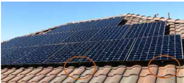
Inside the orange circles are tile replacements.
