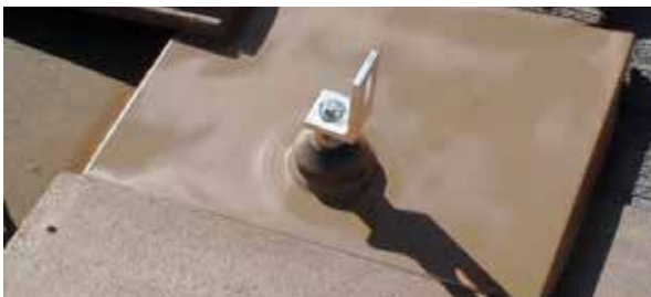
Tile replacement painted to match the roof.
